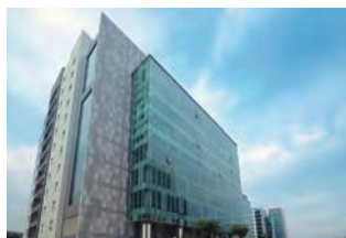
ABS Aircon Engineers Private Ltd. (Indie)
